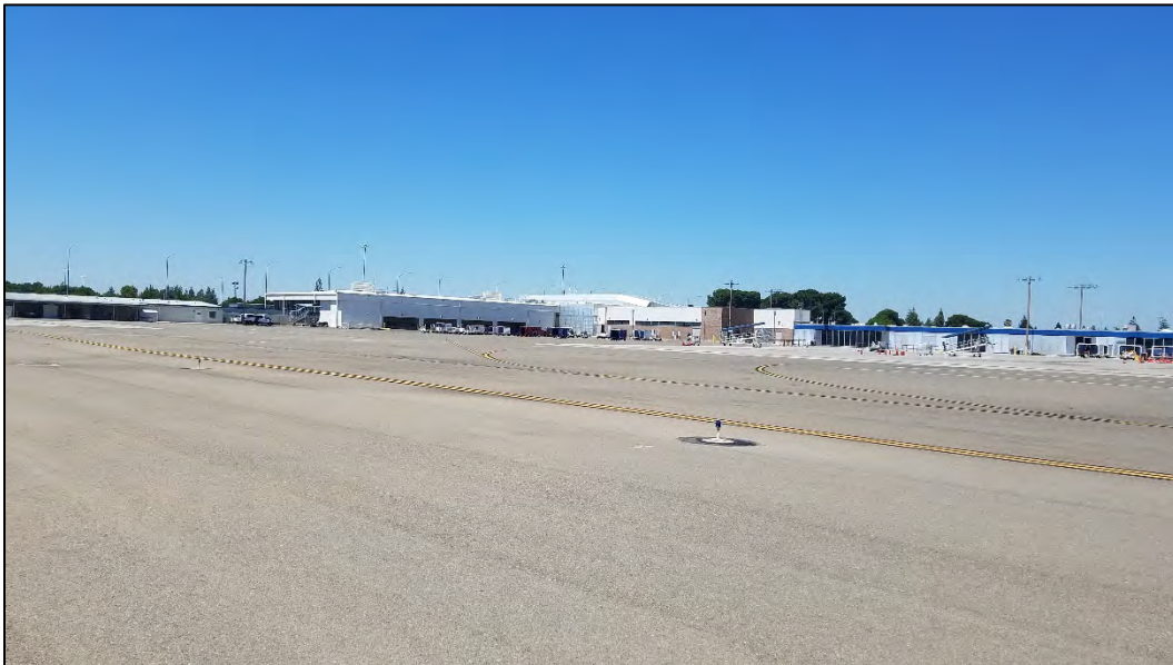
Photo C-6. Representative view of developed conditions in proposed action area. Photo taken May 26, 2020.
