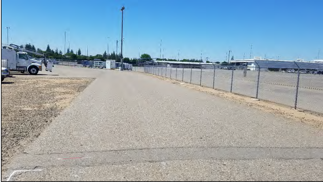
Photo C-5. Representative view of developed conditions in proposed apron expansion area. Photo taken May 26, 2020.
