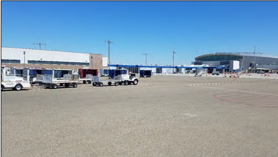
Photo C-2. Representative view of developed conditions in proposed action area. Photo taken May 26, 2020.
