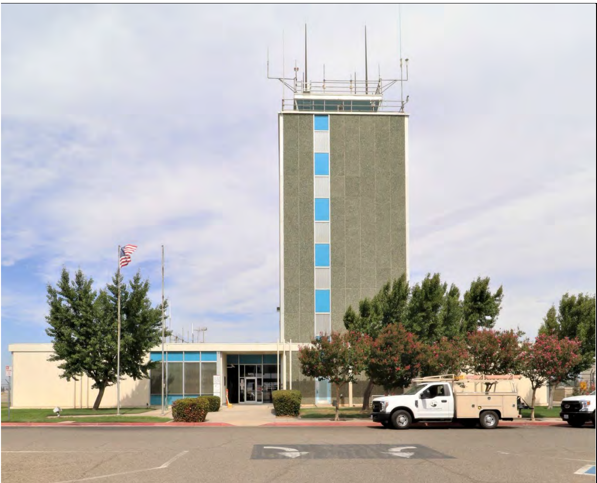
Photo 1: Southwest elevation, view northeast (9/11/23).
