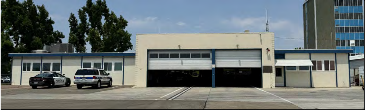
Photo 9: Southeast elevation (faces the Terminal), view northwest (7/30/24).
