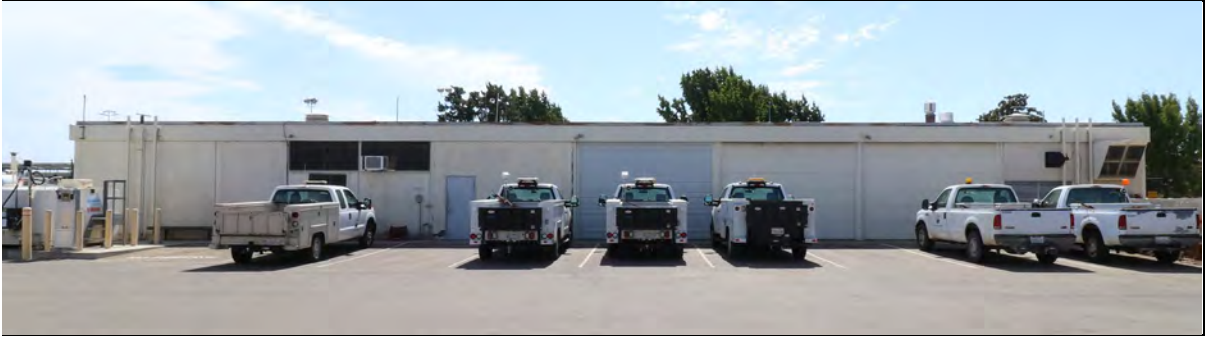
Photo 12: Northeast elevation (faces runway), view southwest (9/11/23).
