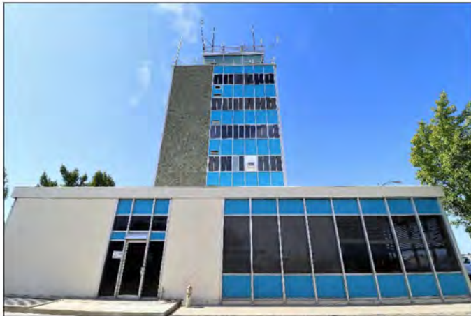
Southeast (side) elevation, view northwest (9/11/23).
