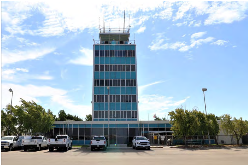
Photo 3: Northeast elevation, view southwest (9/11/23).
