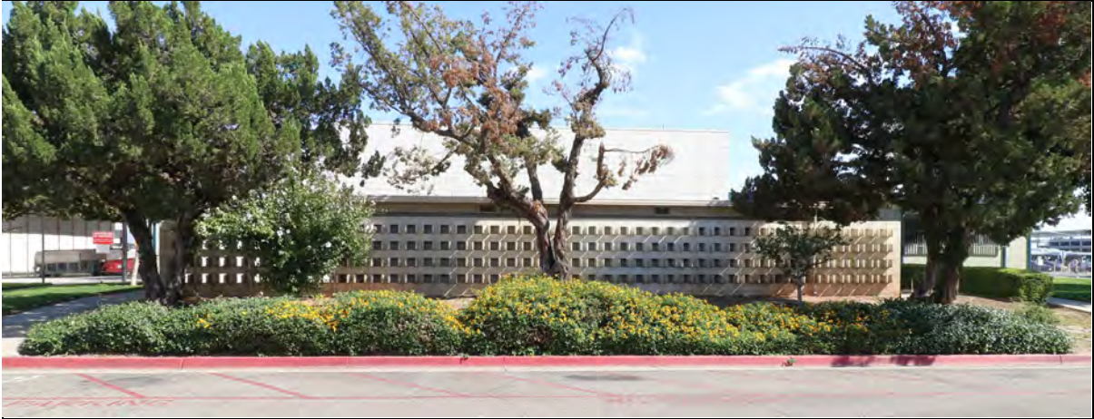
Photo 6: Northwest elevation (adjacent to parking lot), view southeast (9/11/23).
