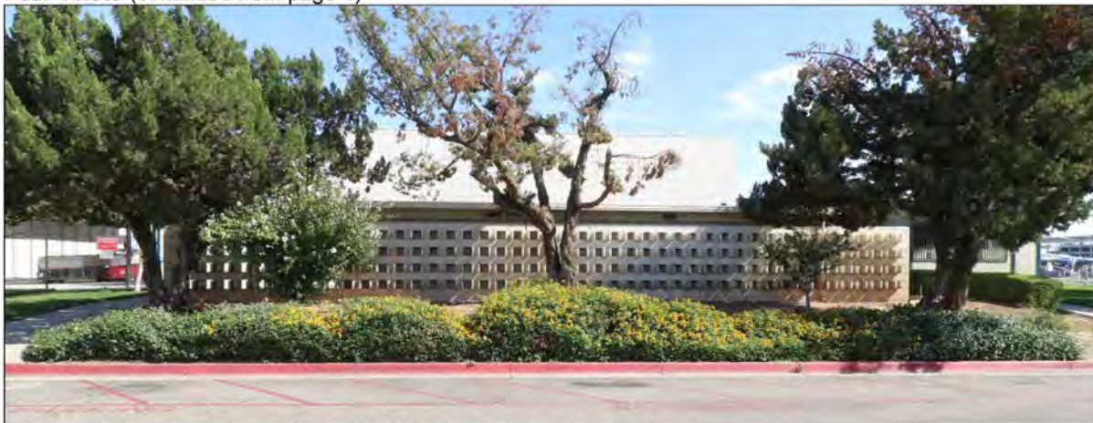
Northwest elevation (adjacent to parking lot), view southeast (9/11/23)
