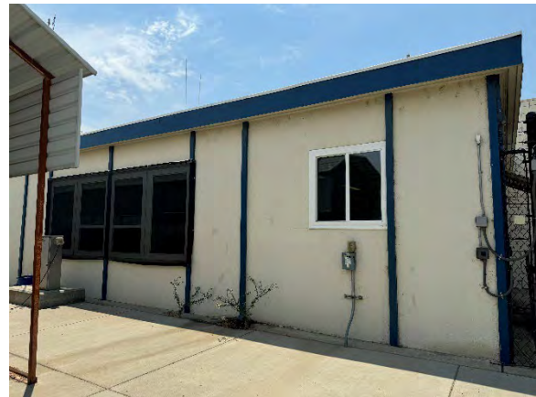
Photo 11: Northeast elevation, view southeast (7/30/24).
