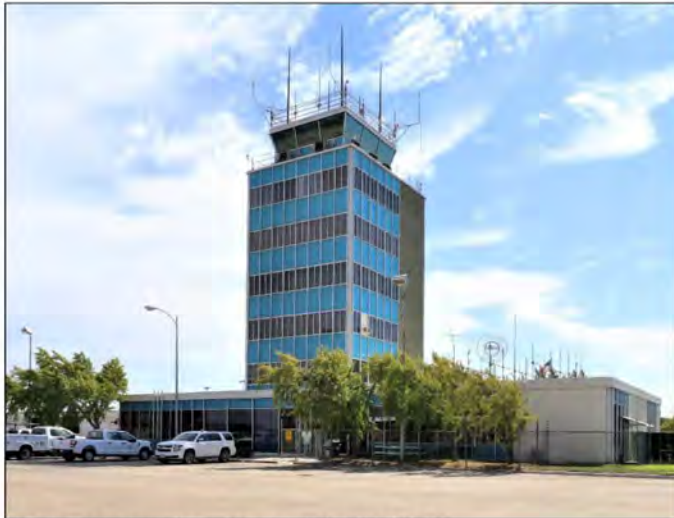
Northeast elevation, view south (9/11/23).
