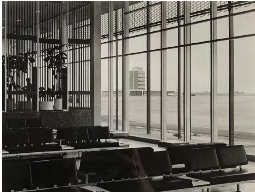
Figure 9: FAT Terminal Interior with View of ATCT (Moore 2023).
