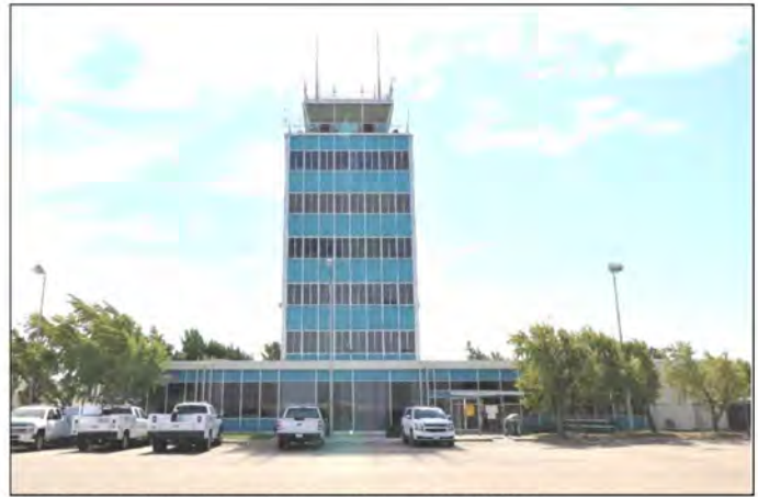
Northeast elevation, view southwest (9/11/23).
