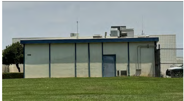
Photo 8: Southwest elevation (facing E. Andersen Avenue), view northeast (7/30/24).
