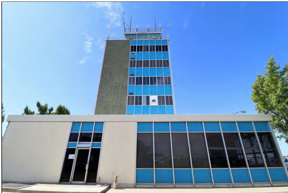
Photo 2: Southeast elevation, view northwest (9/11/23).
