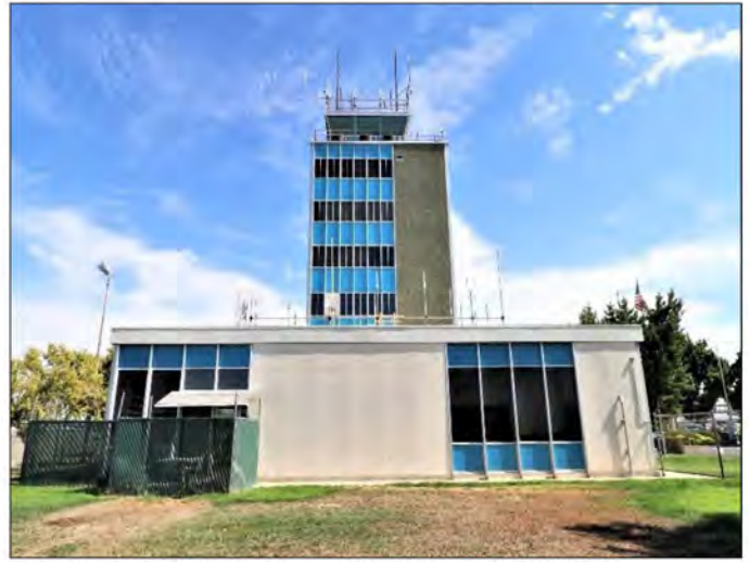
Northwest (side) elevation, view southeast (9/11/23).
