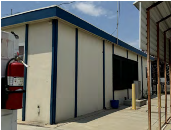
Photo 10: Northeast elevation, view southwest (7/30/24).
